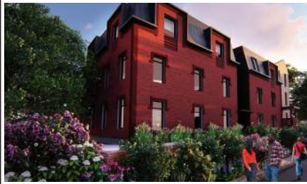
7-UNIT PASSIVE HOUSE
