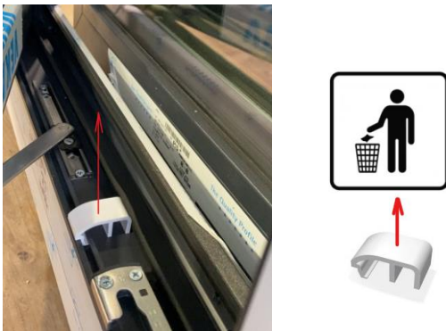
Fig. 7. Sash spacer shims:
