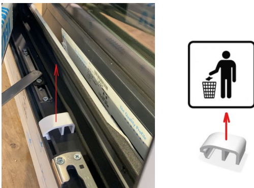
Fig. 7. Sash spacer shims:
